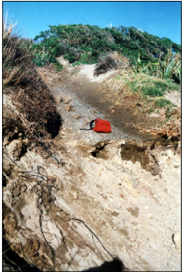
PHOTOGRAPH 9: Foredune erosion, exacerbated by access from coastal track, between Raumati and Whareroa Stream. Access could be discouraged by flax planting at top picture.
