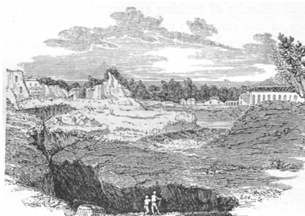
Deep fissure, near Polistena, caused by the earthquake of 1783.
