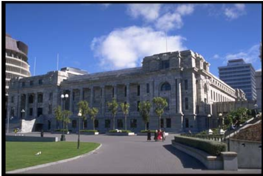
Figure 2a: NZ Parliament Buildings seismically isolated using Lead Rubber Bearings
