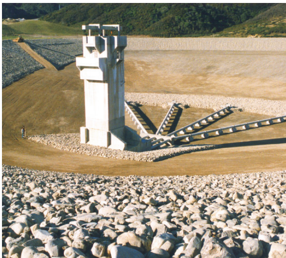
Building the Te Marua storage lakes, 1987
