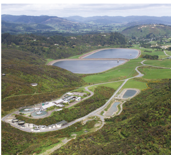
Aerial view of Te Marua storage lakes and water treatment plant
