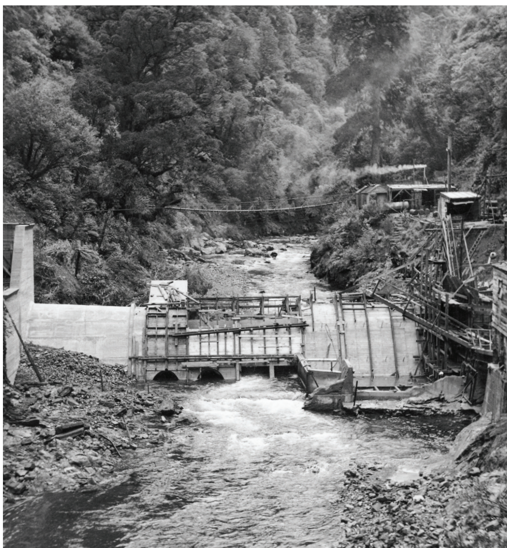
Kaitoke Weir construction
