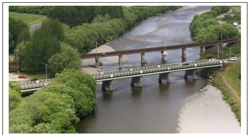
Silverstream Bridge is a key river crossing for the main (green) pipeline from Te Marua
