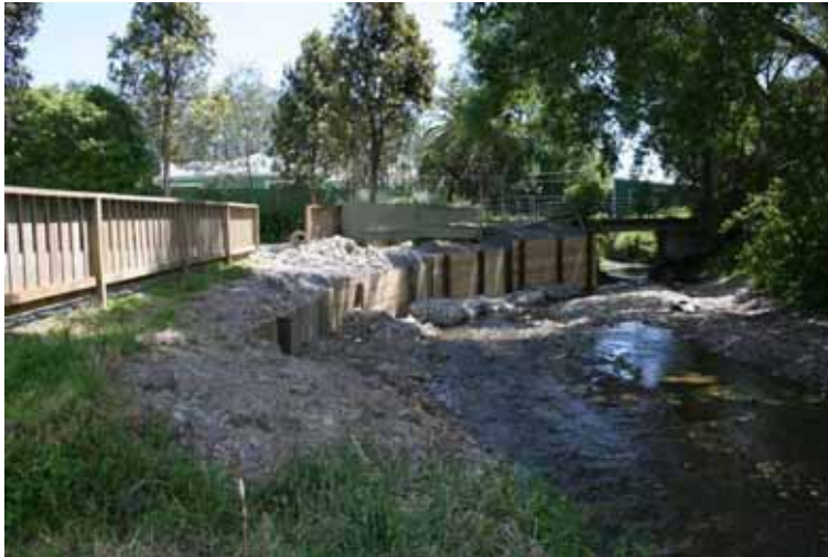
A timber wall in Wharemauku Stream
