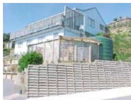
Figure 3.8: Water Storage Tanks
