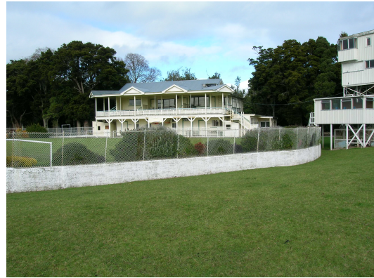
Tauherenikau Racecourse complex with the bush in the background
