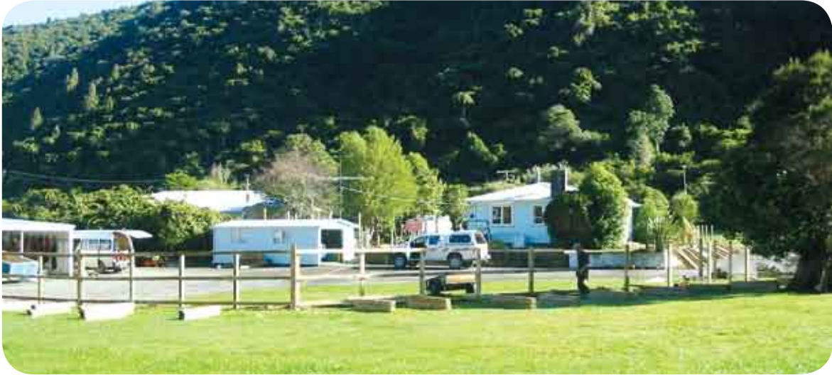
Building a new fence around the Rangers' houses and storage area
