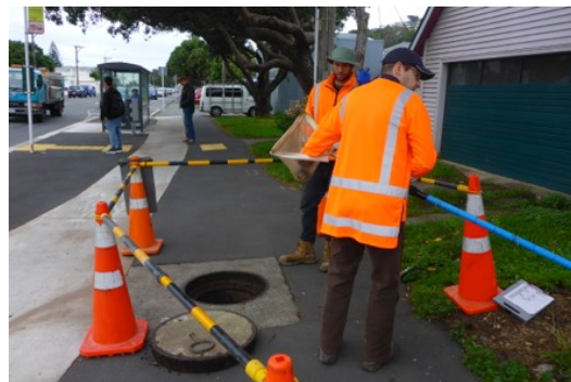
Pae Kawakawa Stream manhole on footpath
