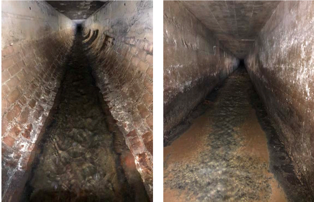
Figure 22 Long, homogenous zones of high water velocities at the Waipapa Stream site (left) and The Parade – Dover St site in the Pae Kawakawa catchment (right).
