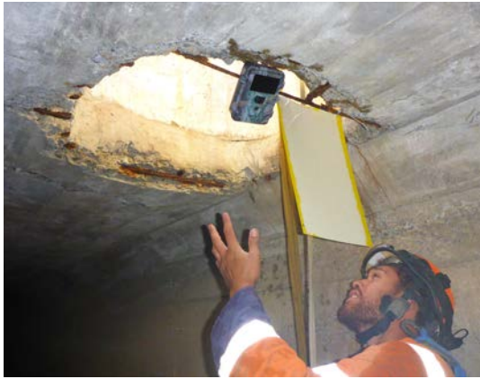
Camera and sticky trap attached to reinforcing steel
