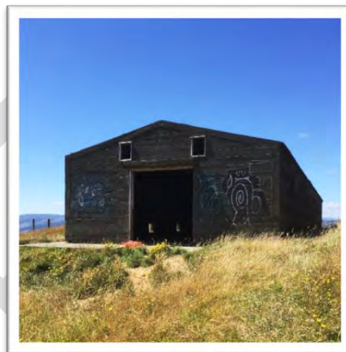
The interesting and unique Belmont Bunkers have the potential to be a significant destination, achieved with simply by opening access to the large car park at the top of Hill Road from where an easy flat 2km circuit walk takes in 17 bunkers and the row of eight ‘magazines’ with stunning views.
