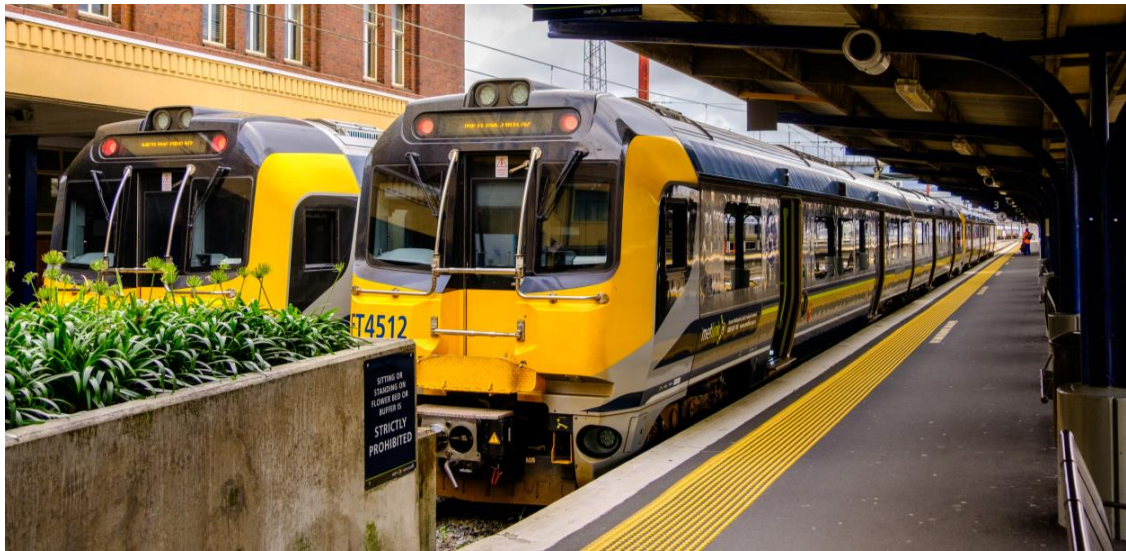
Wellington Station is a key hub for travel to and from our region and beyond
