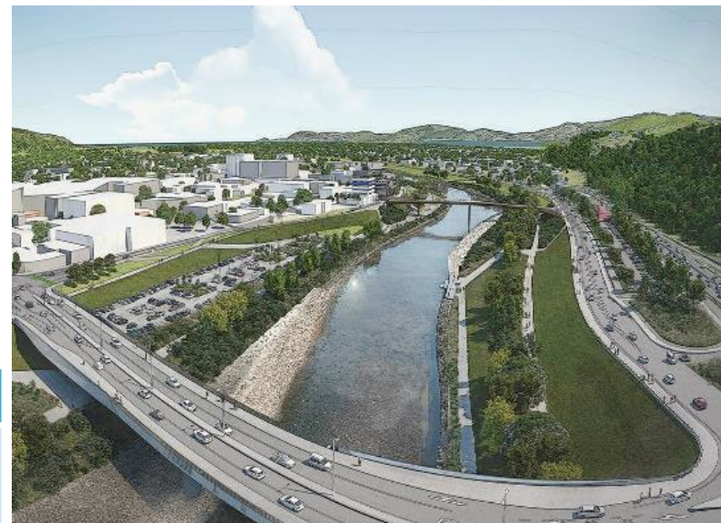
Aerial view of the new Melling bridge and pedestrian/cycle bridge connecting to the relocated Melling train station ( draft impression, subject to change ).
