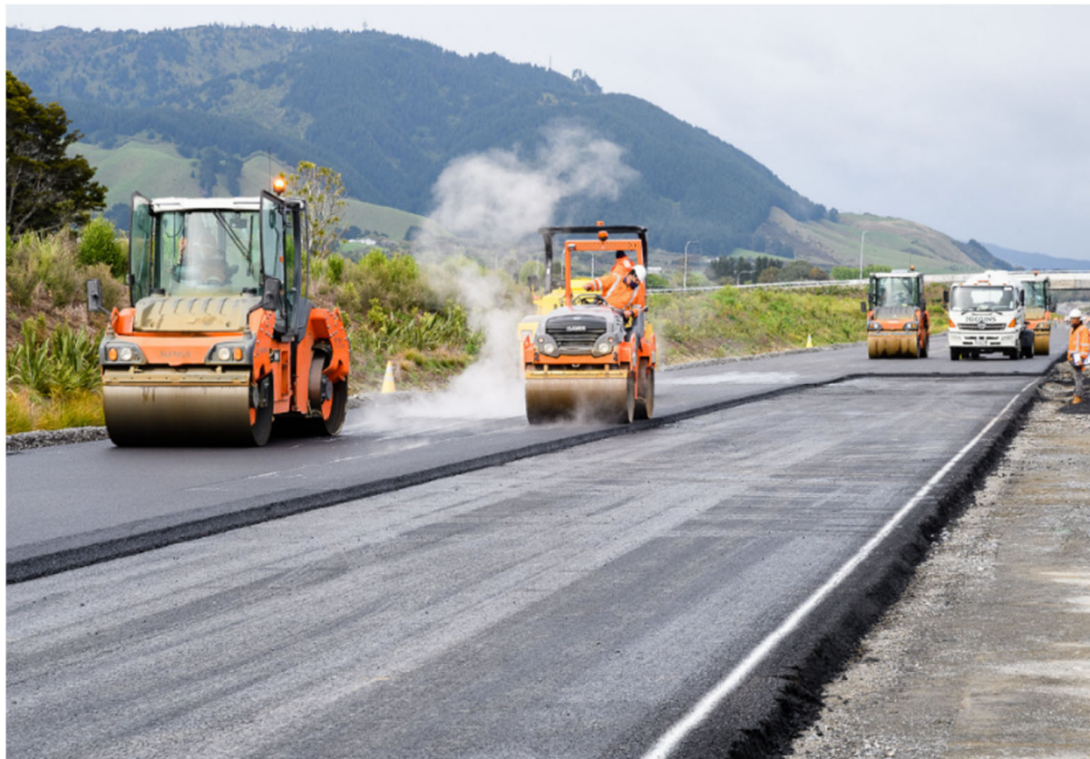
Pavement works on southbound lanes, near Te Horo
