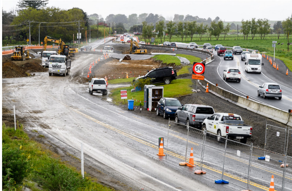
Northern diversion on SH1, allowing tie-in works to commence
