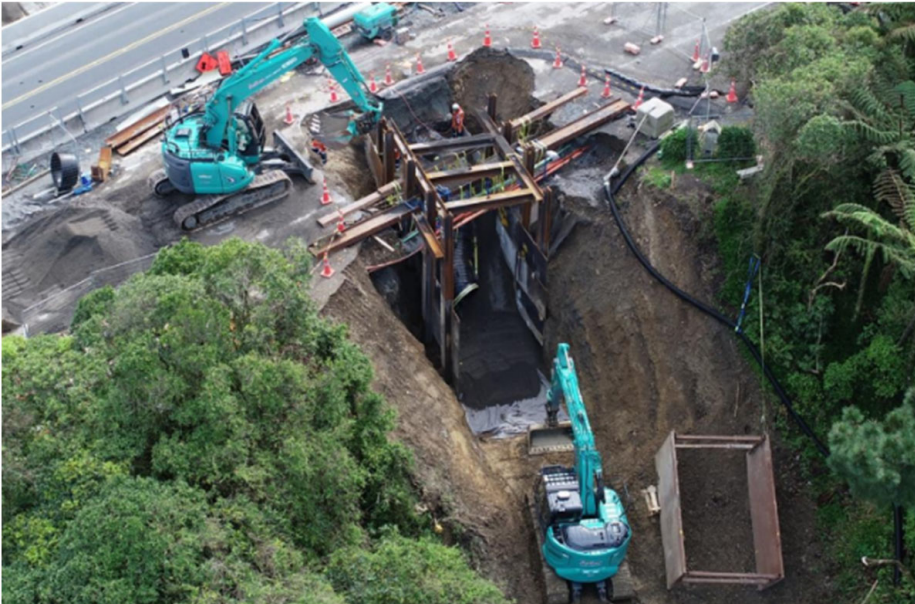
Drone image of culvert installation, near Hugh Duncan St
