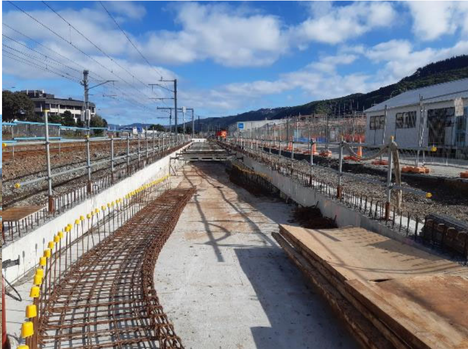
Ramp at Petone underpass taking shape
