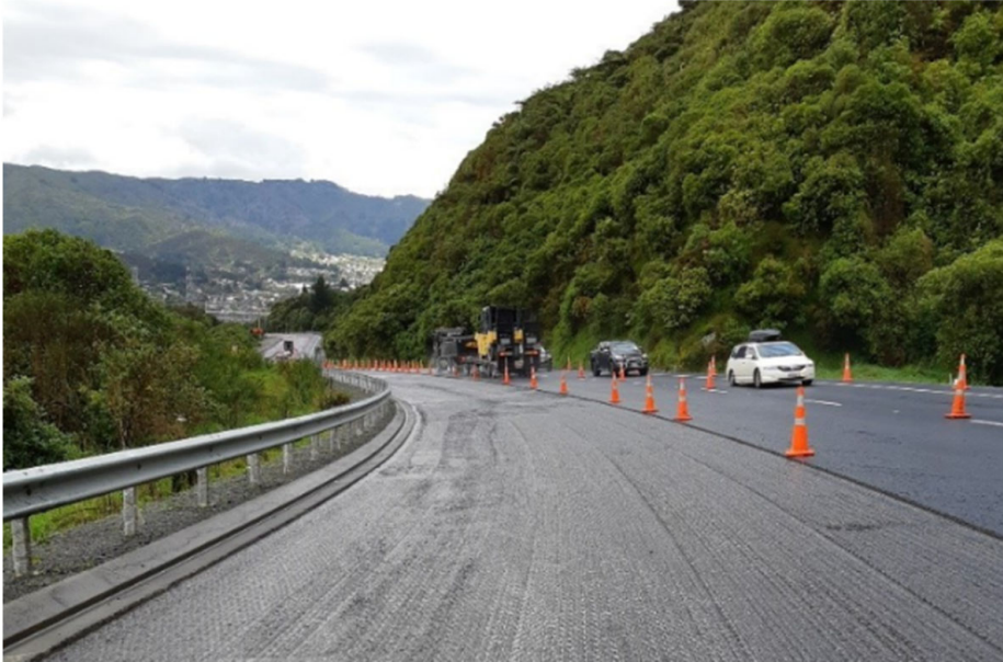
Surfacing works – looking east towards Hutt Valley
