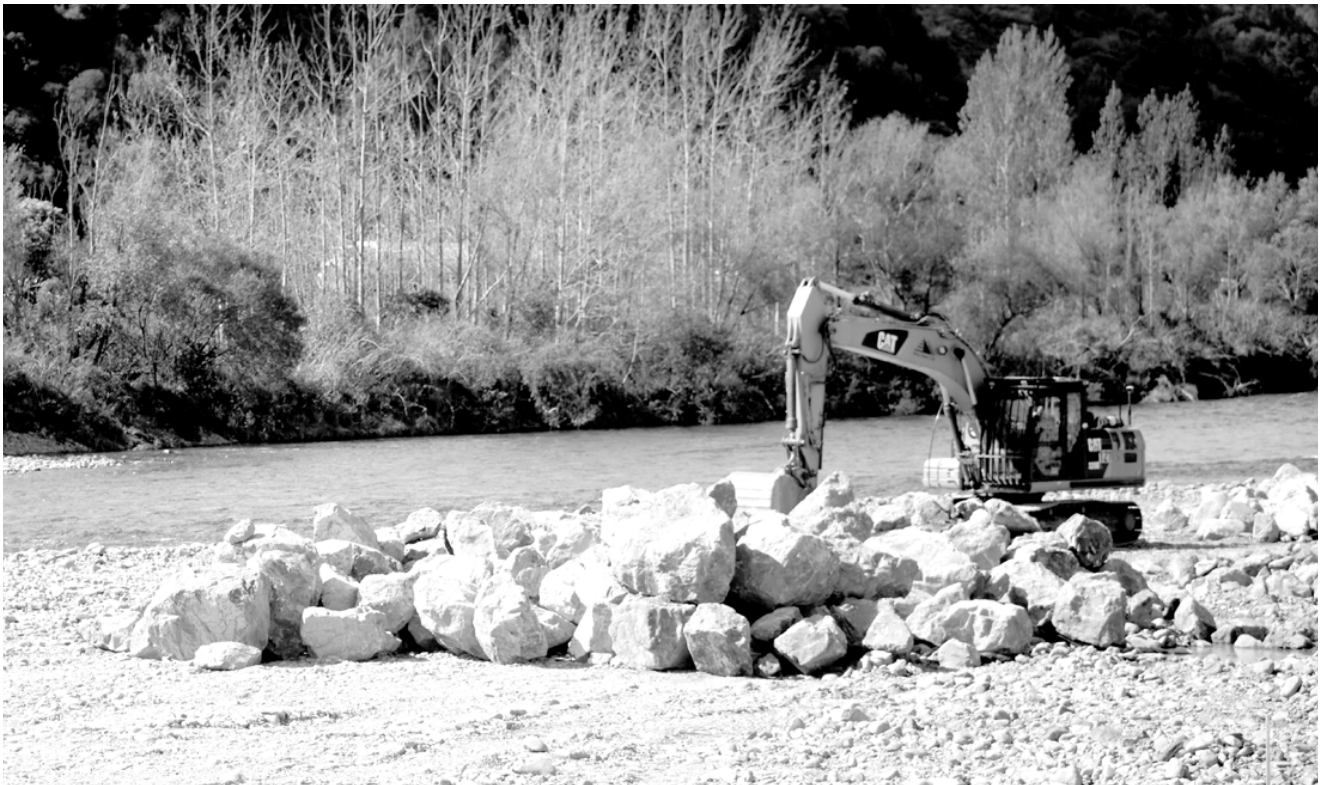
Flood protection work happening on the Hutt River
