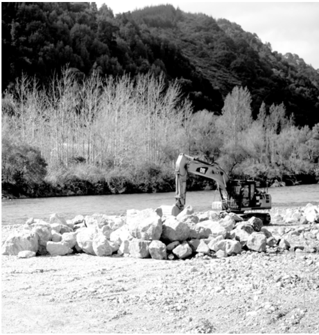
Flood protection work happening on the Hutt River
