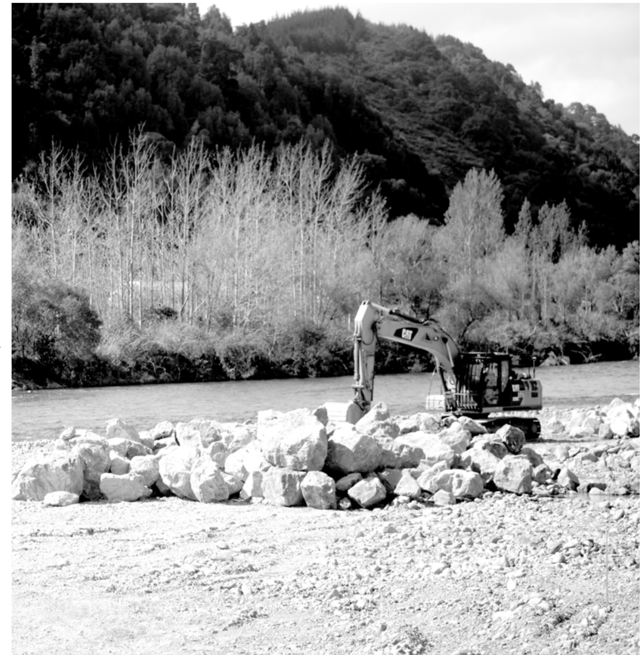
Flood protection work happening on the Hutt River
