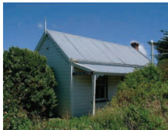
Taylor Stace cottage, Pauatahanui - classified as Category 1 on the Historic Places Trust Register and therefore a 'regionally significant' heritage item in the Regional Policy Statement. Photo: R. McClean, NZHPT, 2004.
