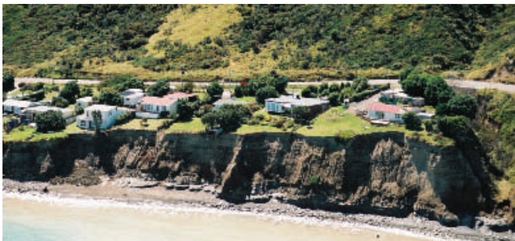
Te Kōpi, Palliser Bay, 2002. Coastal erosion is a continuing problem for settlements and the road along this stretch of coast.
