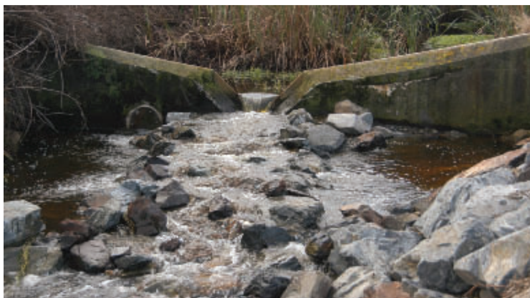
The Taupo Stream fish pass, installed in 2005, helps native fish like inanga and giant kokopu get upstream into Taupo Swamp once again.
