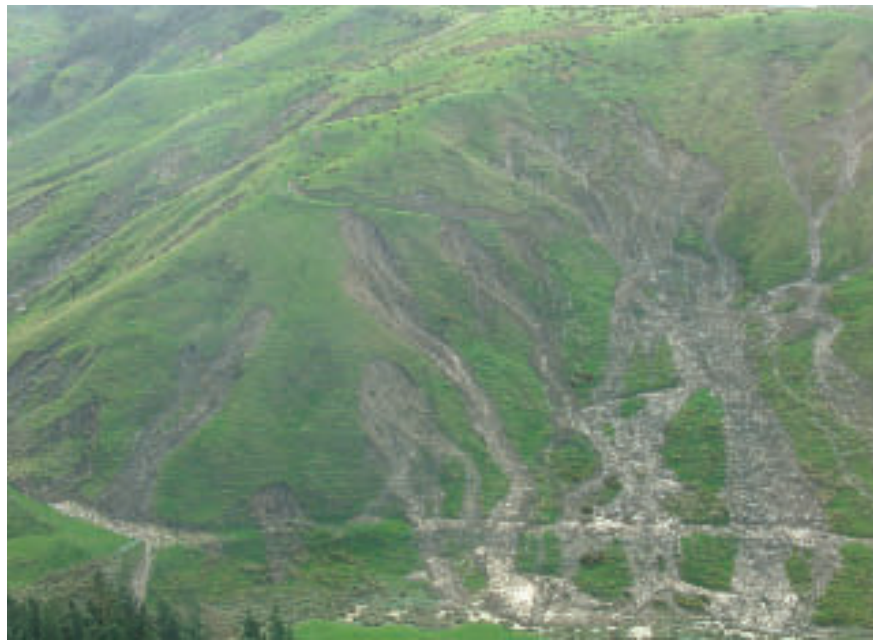
Shallow soil slides at Castlepoint Station in the eastern Wairarapa hill country, triggered by intense rainfall in March 2005. Photo: Masterton District Council.
