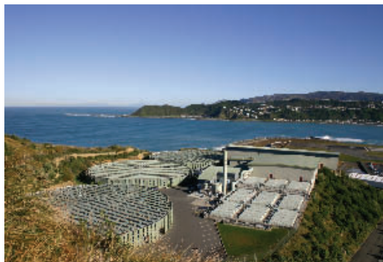
Wellington City Council’s sewage treatment plant at Moa Point near Wellington serves a population of about 130,000. The sewage is treated by screens, aerated tanks, bioreactors, clarifiers and finally ultra violet light for disinfection. The treated effluent is discharged from a 1.8 km outfall into Cook Strait.
