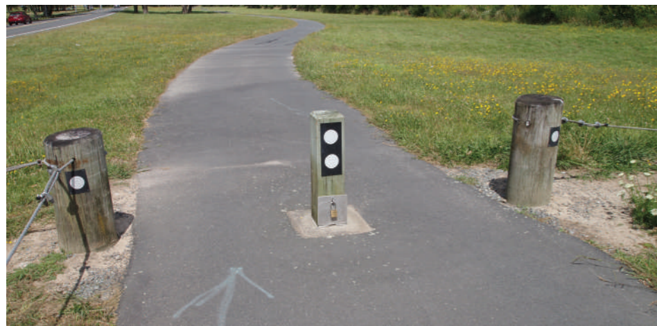
TYPICAL SQUARE REMOVABLE TIMBER BOLLARD
