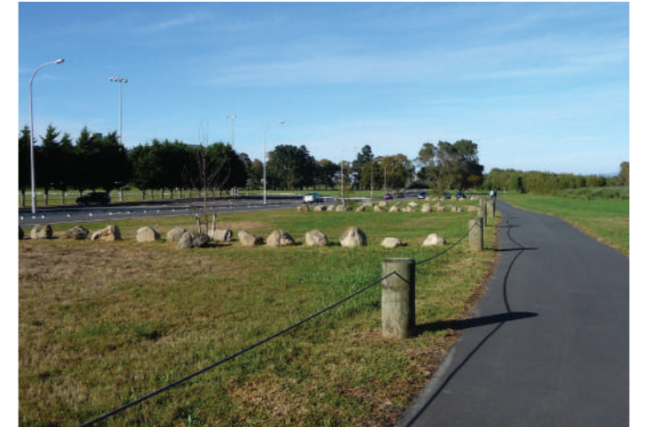
Existing simple bollards with chain and rock edging
