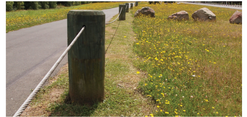
TYPICAL TIMBER BOLLARD WITH WIRE ROPE
