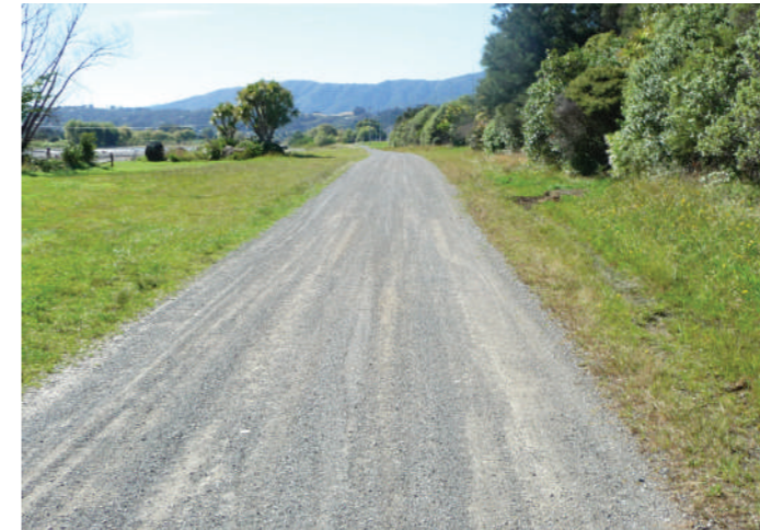
Soft surfacing for vehicle access
