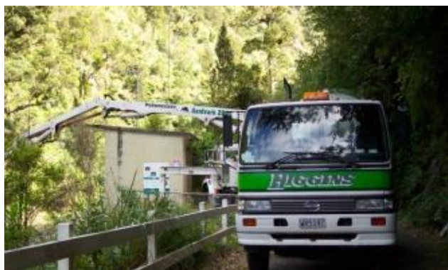
Maintenance activities at Kaitoke Weir. The threat of contamination from vehicles entering the water collection areas is actively managed via means such as standard operating procedures and works contract conditions
