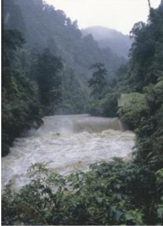
Hutt River in flood at Kaitoke Weir in 1995 making it almost invisible (refer other photos). The very steep slopes of the Western and Eastern Hutt Rivers create fast water flows and the potential for significant erosion, particularly if overall vegetation health is not maintained. Flood events deliver a much higher sediment load to be filtered for drinking water via the water treatment plants.
