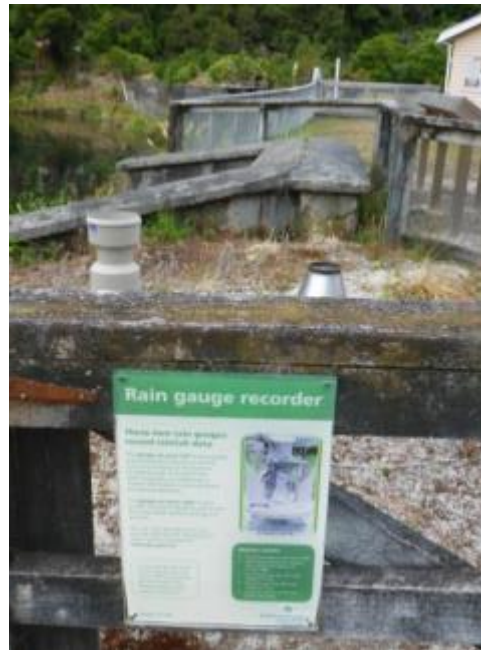
Rain gauge recorder at the Waterworks /Lower Dam, Wainuiomata Recreation Area which adjoins the Wainuiomata Water Collection Area
