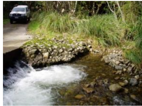
The design of the Sinclair Creek culvert and ford run off encompass embedded rocks to capture sediment runoff to the creek becoming mossy over time
