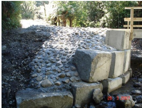
The design of the Sinclair Creek culvert and ford run off encompass embedded rocks to capture sediment runoff to the creek becoming mossy over time
