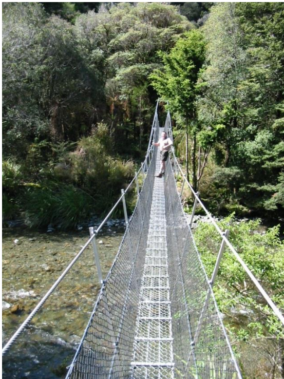
A suspension bridge at Hutt Forks minimises risks from water contamination via river crossings and provides access to the Quoin Ridge route
