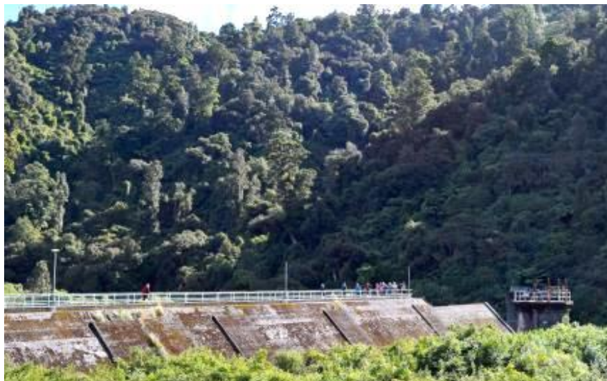
Guided walking tour viewing Morton Dam. Construction of this dam was completed in 1911 and it was decommissioned and superseded by the Te Marua lakes scheme in 1988. The dam is historically significant because of its form of construction which is unusual in New Zealand; reinforced concrete made in sections of slab and buttresses.
