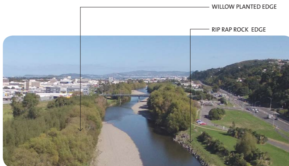
FIGURE 10 River bank edge protection treatments - rock or willow protection
