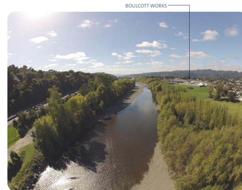
FIGURE 9 Boulcott area works
