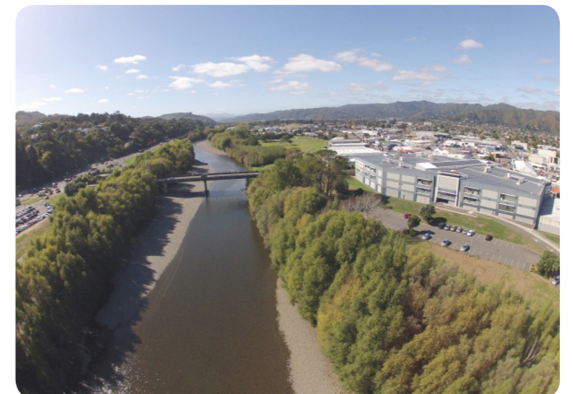
FIGURE 7 Shows the proximity of development to the stopbank edges
