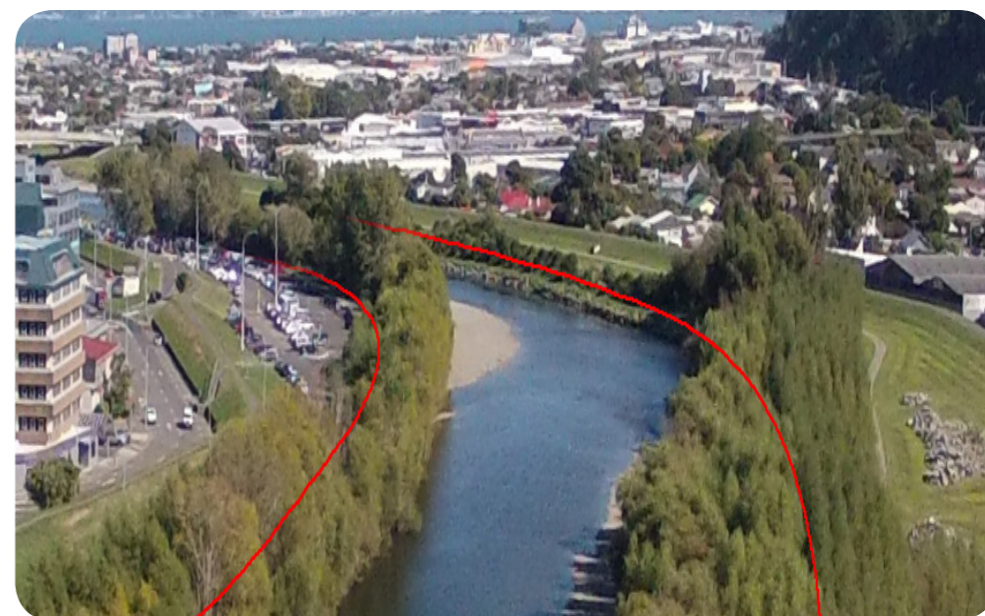
FIGURE 12b Channel widening past the city centre area
