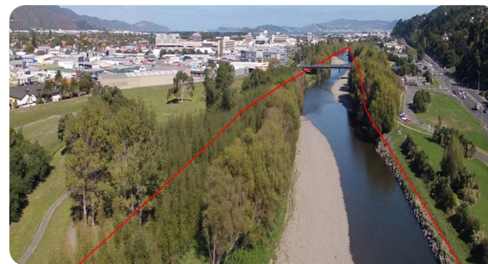
FIGURE 12a Channel widening from upstream and past of Melling Bridge
