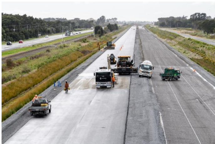
View from Te Horo overbridge – Bridge 8
