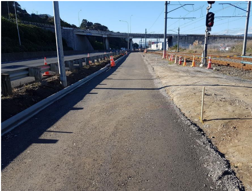
Kerb and Channel – main alignment
