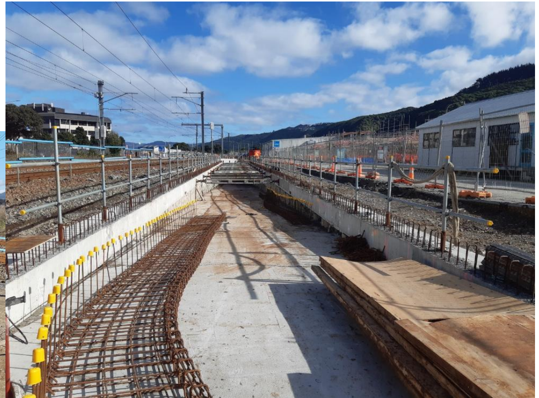
Ramp at Petone underpass taking shape
