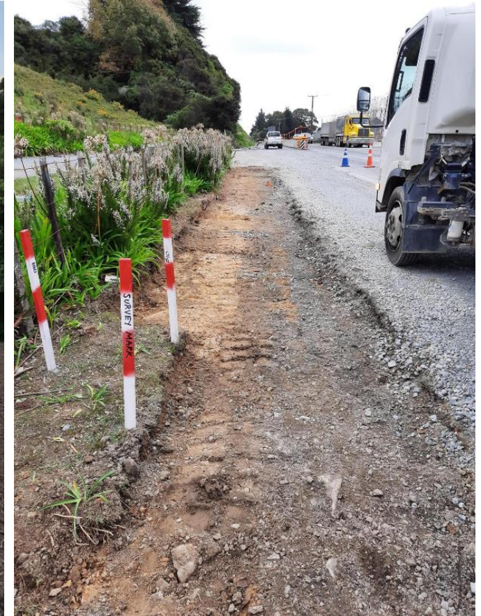
Surfacing preparation works
