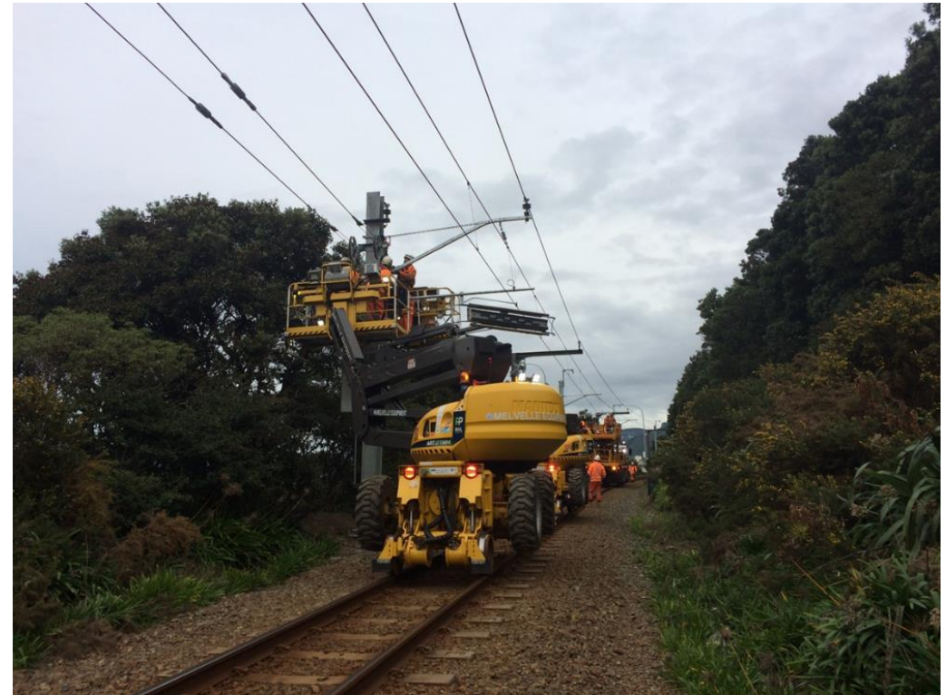
OHLE wiring run at Queens Birthday BOL
