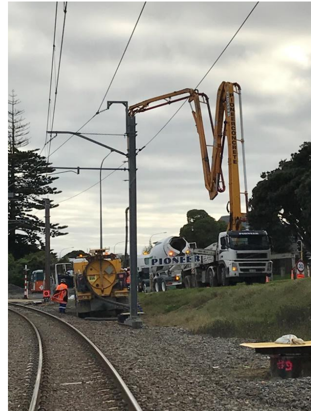
Concreting new pile at Plimmerton to allow OHLE to be realigned
