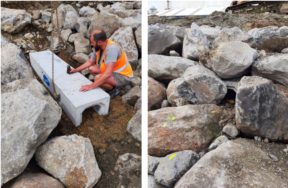
Figure 1: Port Road site penguin 'hotel' - being placed and showing entrance
