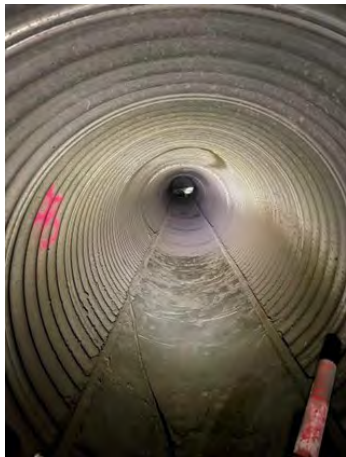
Culvert and outlet remediation
