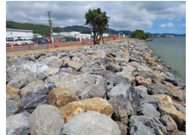
Revetment construction
