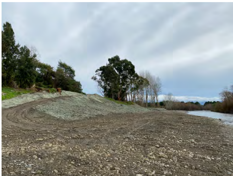
Figure 31: Ruamāhanga River - site of groyne construction
