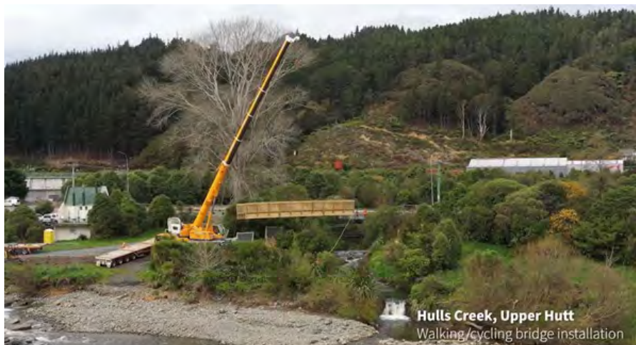
Figure 4: Hulls Creek Bridge installation
