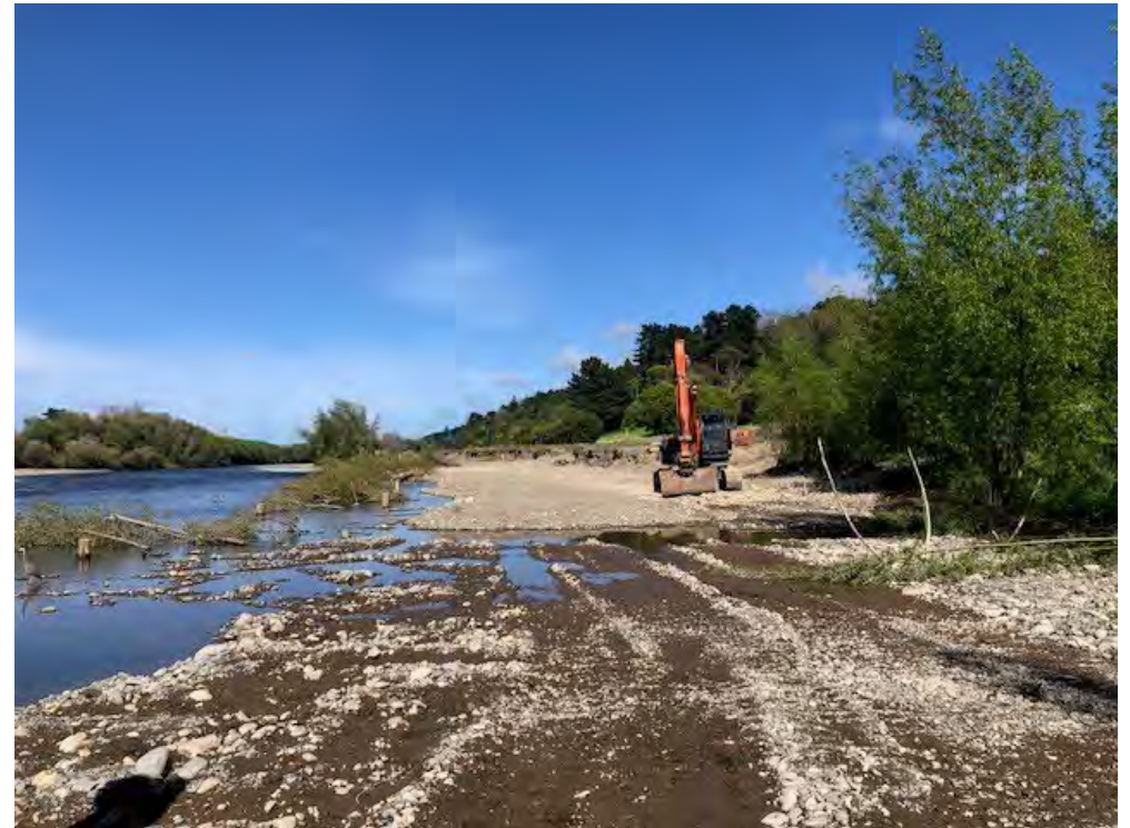
Photograph: Construction of debris fences along Te Awa Kairangi/Hutt River
