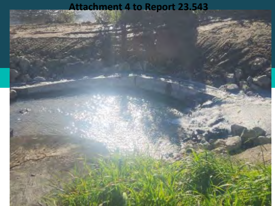
Weir repair and fish passage construction
