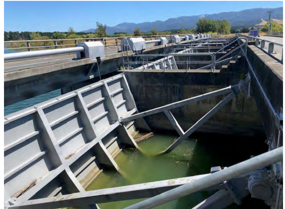
Photograph: Geoffrey Blundell Barrage Gates
