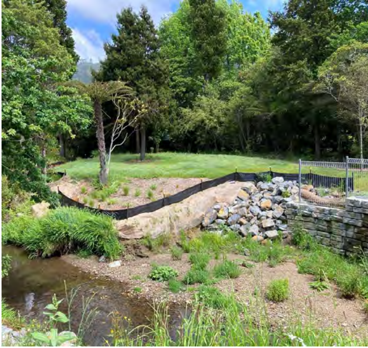
Figure 6: Willow Park vegetation clearance and setup for the stream bank upgrades (photo credit: GHD)
