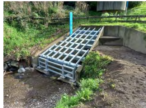
Culvert and outlet remediation
