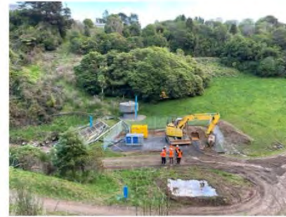
Seton Nossiter Park culvert improvements advancing well
