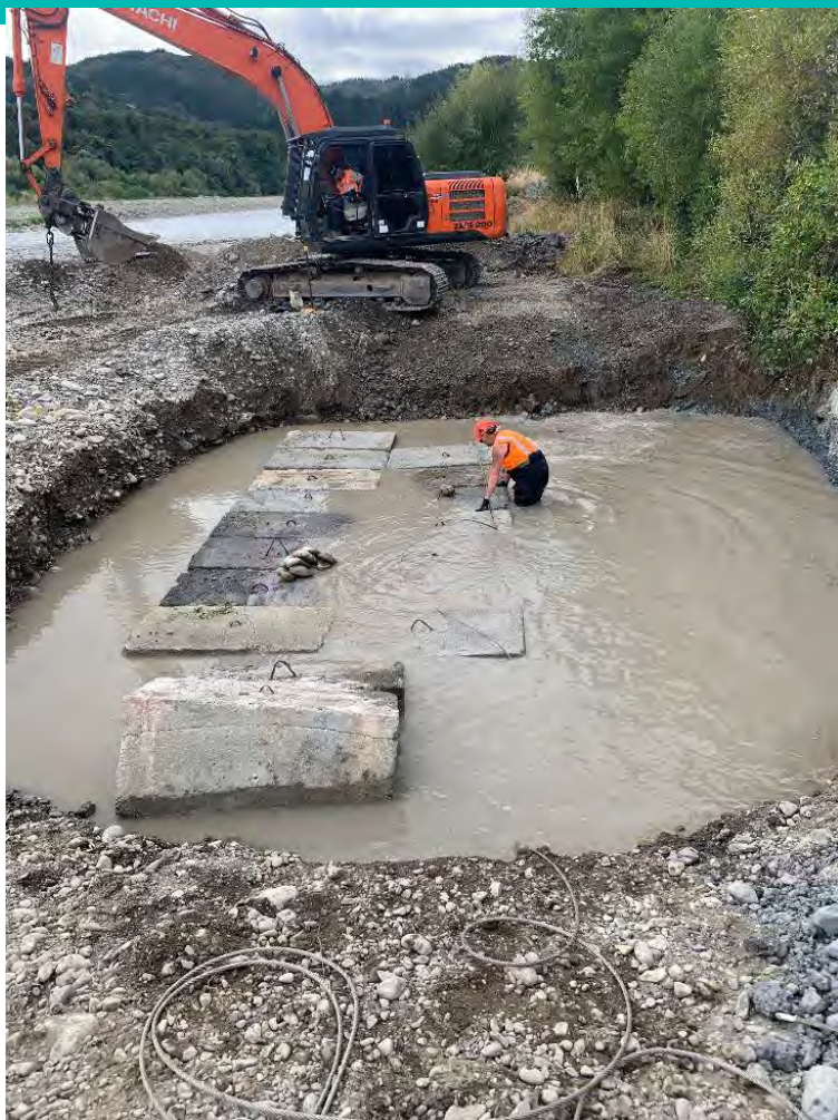
Building rock groynes at Whakatikei
