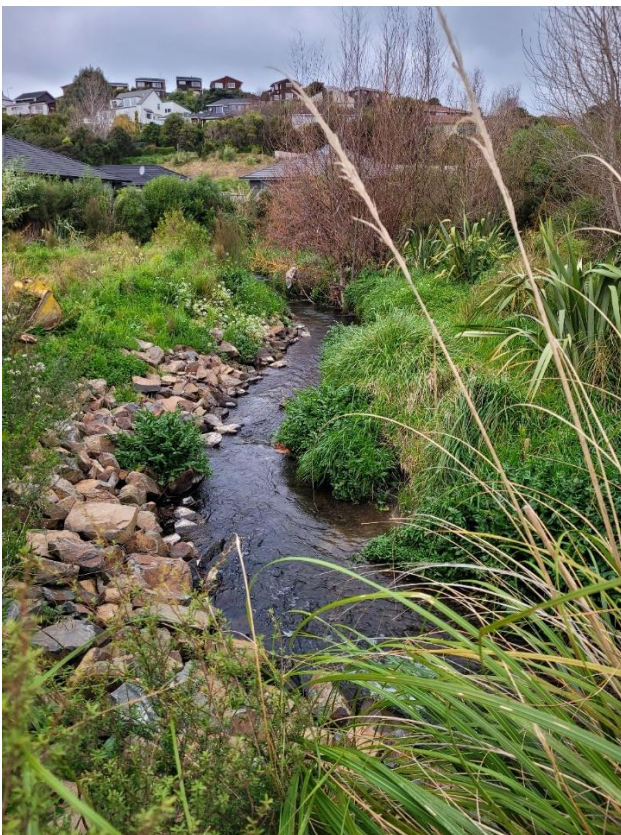
Figure 3: Rock lining in Wai-o-Hata/Duck Creek catchment to protect subdivision. Source: Natasha Petrove, DOC Technical Advisor Freshwater, based in Wellington.
