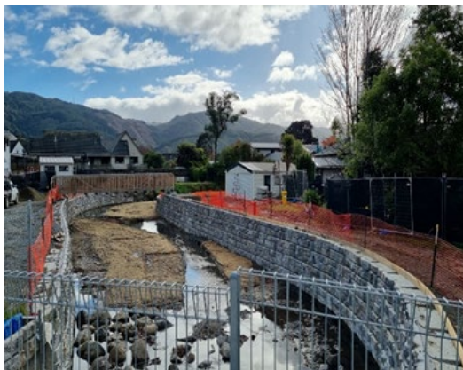
Figure 1 Looking downstream from Sunbrae Dr. towards pedestrian bridge (photo credit: GHD)
