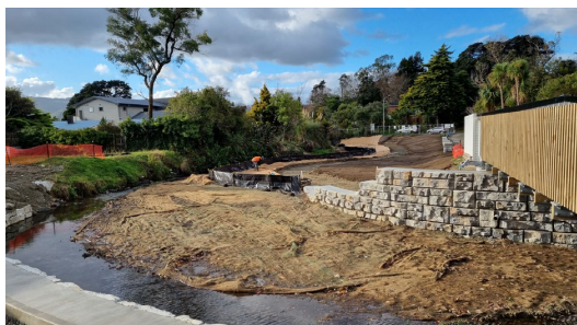
Figure 3 Pinehaven Stream siteworks looking downstream from pedestrian bridge (photo credit: GHD)
