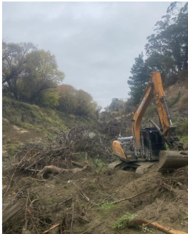
Figure 4: Whareama River – blockage removal commenced
