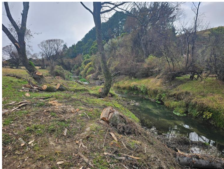
Figure 2: Kopuaranga River – post blockage removal
