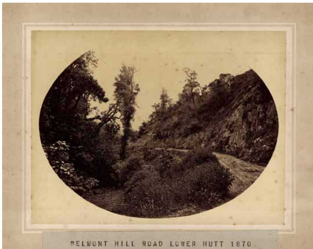
A Section of the Completed Belmont-Pauatahanui Road, 1870: Alexander Turnbull Library, PA Coll-1574-17
